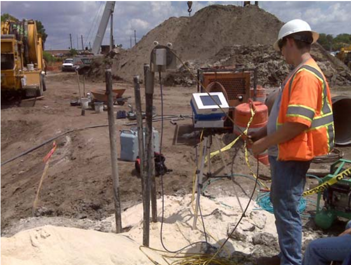
Thermal Integrity Profiling for FDOT, Tampa (Probe version).
